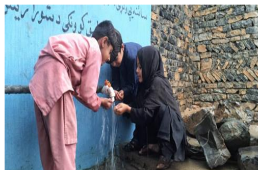
Installation WASH facilities at Sekandar khial village high school, Ahamad Khial district, Paktika Province. © UNICEF
